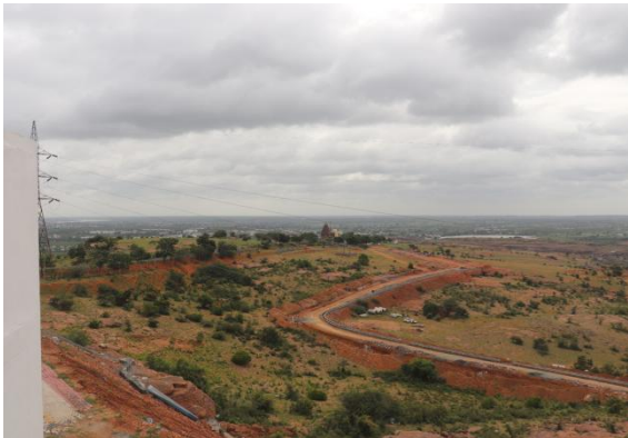
Bulk Services – Construction of Roads
