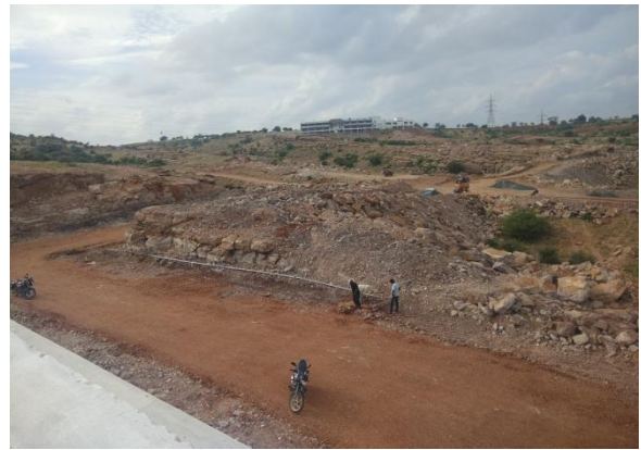
Bulk Services – Construction of Roads
