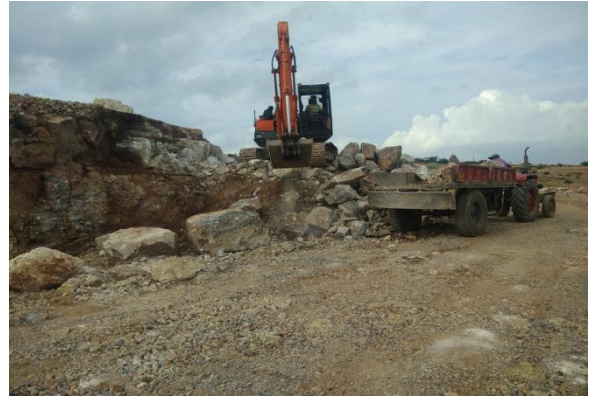
Bulk Services – Construction of Roads
