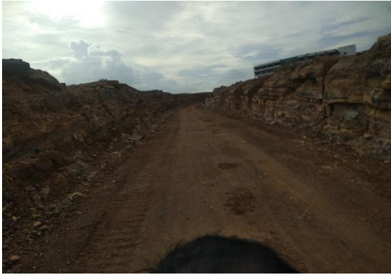
Bulk Services – Construction of Roads
