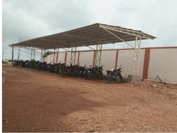
Parking Shed at Administration Block
